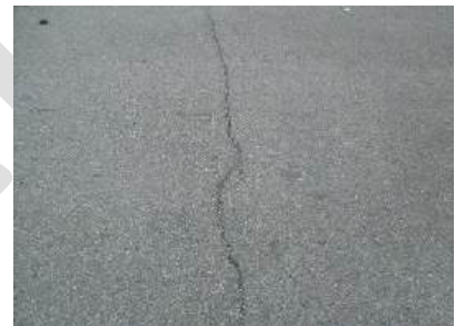
Figure 12: Longitudinal Cracking
