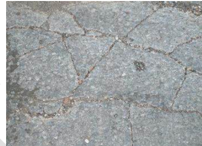
Figure 11: Fatigue Cracking
